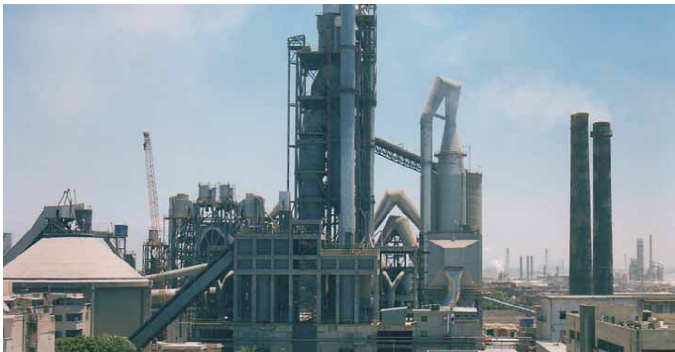
Alexandria plant, Egypt
