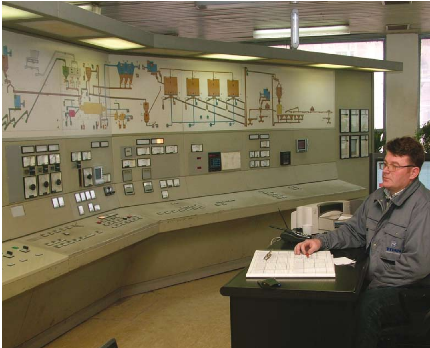
Control centre, Kosjeric plant - Serbia, 2005
