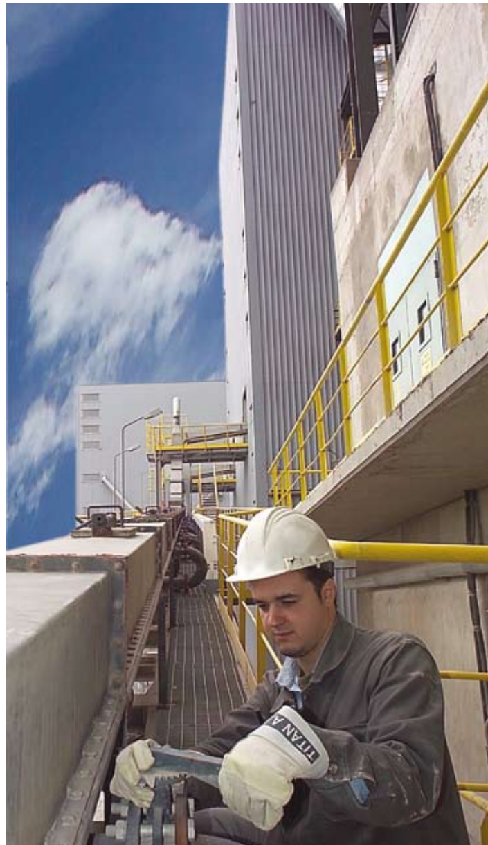
Thessaloniki plant - Greece, 2005
