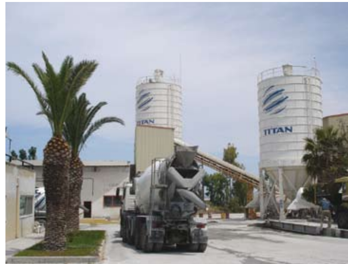
Concrete plant, Rhodes - Greece
