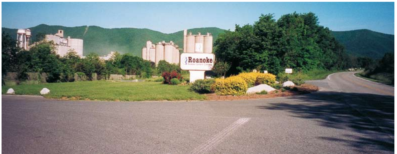
The Roanoke plant – USA, 2005
