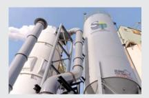
alternative fuels. The Pennsuco plant now produces its own kiln fuel at a new Processed Engineered Fuel (PEF) facility, which will offset the plant's existing fossil fuel usage by up to 30% while diverting municipal waste from landfill.
