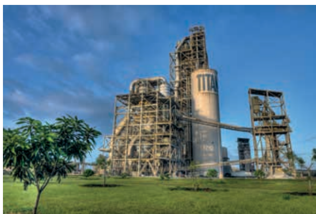
Pennsuco cement plant, USA
