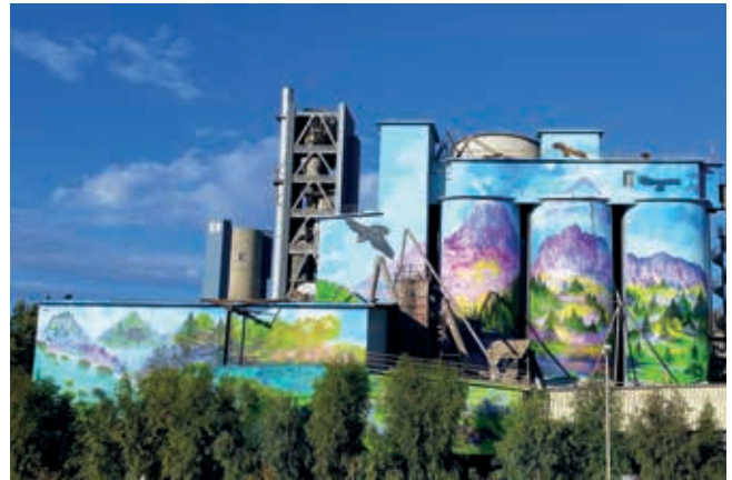
Thessaloniki cement plant, Greece
