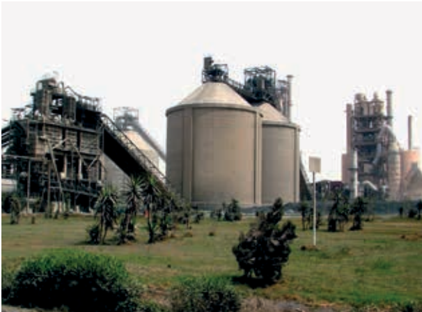
Beni Suef cement plant, Egypt
