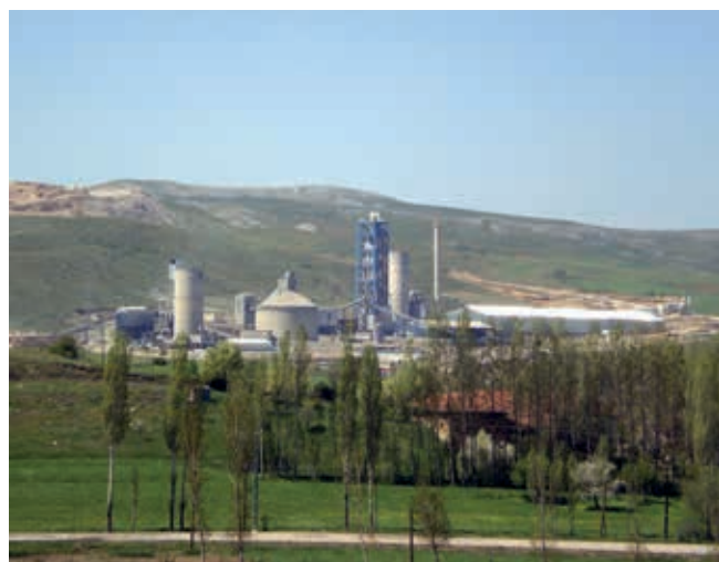
Tokat cement plant, Turkey
