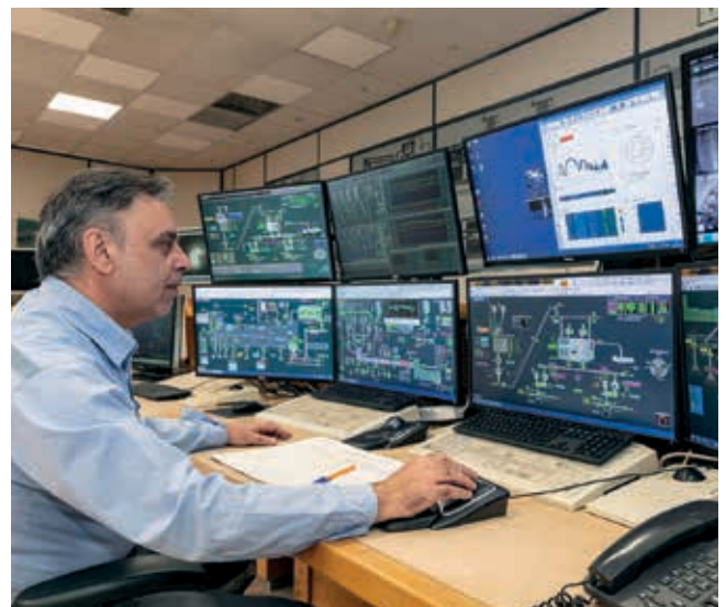
Kamari cement plant, Greece
