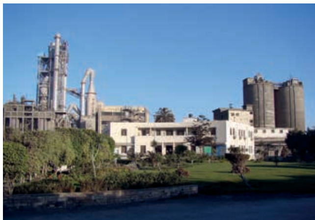
Alexandria cement plant, Egypt
