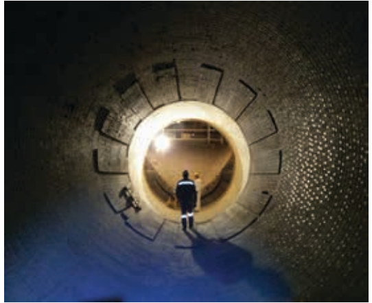
Kamari cement plant, Greece
